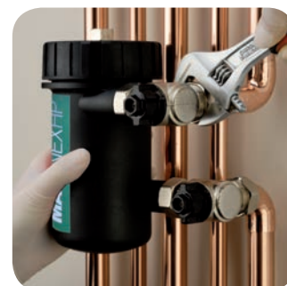
Fig. 3 - Tighten the compression joints
